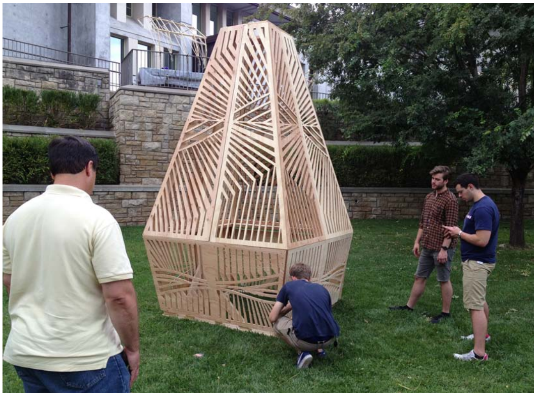
Figure 6. Eternal Frame Sculpture being installed on site
