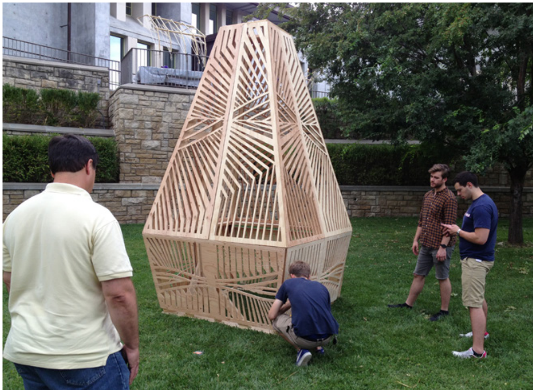
Figure 6. Eternal Frame Sculpture being installed on site
