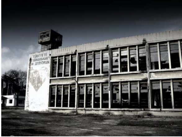
Figure 4. Nazilli Sümerbank Factory building
